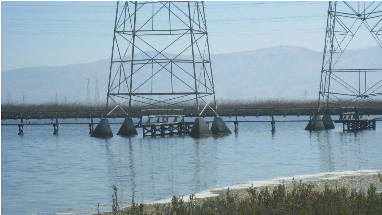
Figure 4.14. PG&E Electrical Transmission Towers and Footings in Pond A2W.
