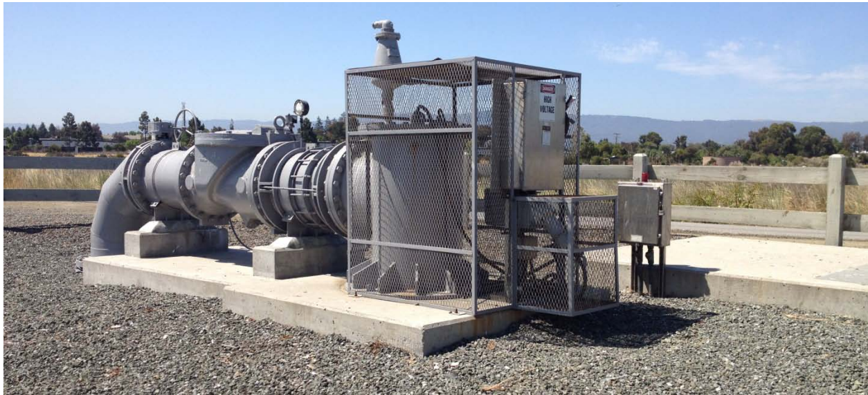
Figure 3. Photo of the Sailing Lake Pump Station Wet Well with the Valve Vault in the background to the right.
