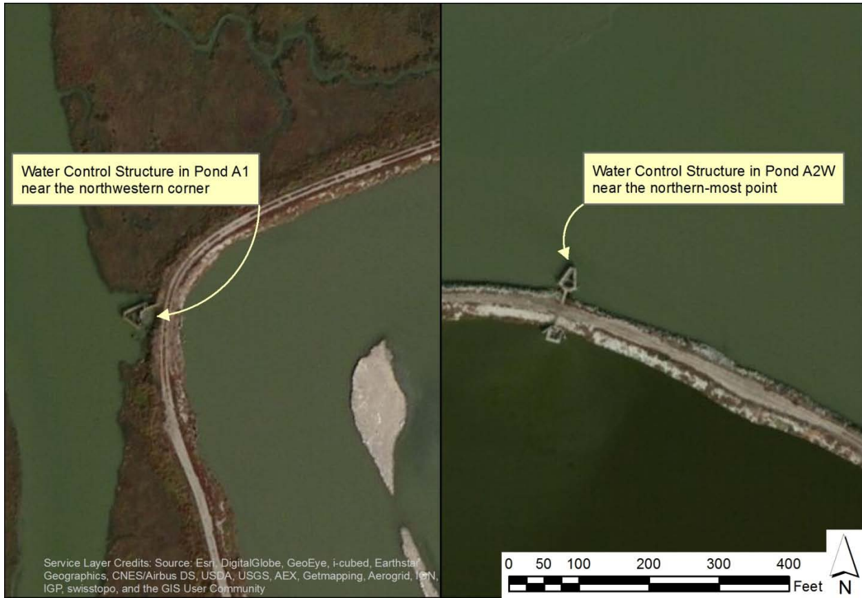
Figure 4.1. Aerial View of Water Control Structures
