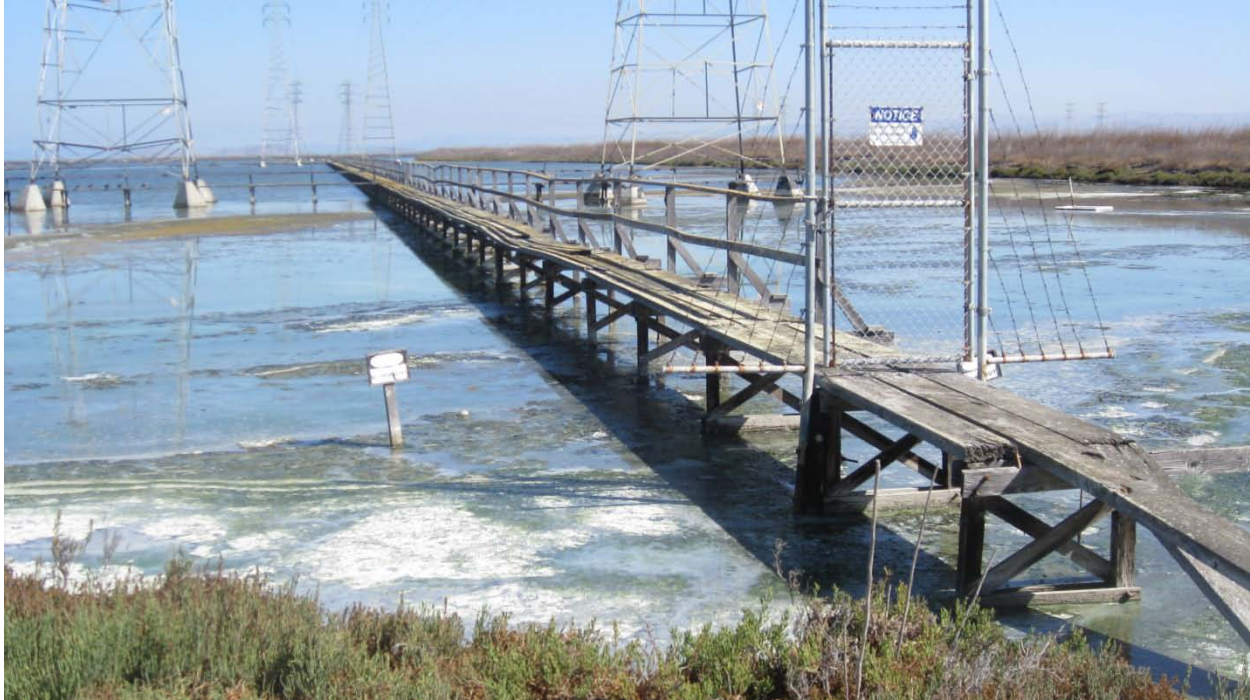
Figure 4.15. PG&E Access Boardwalks in Pond A2W.
